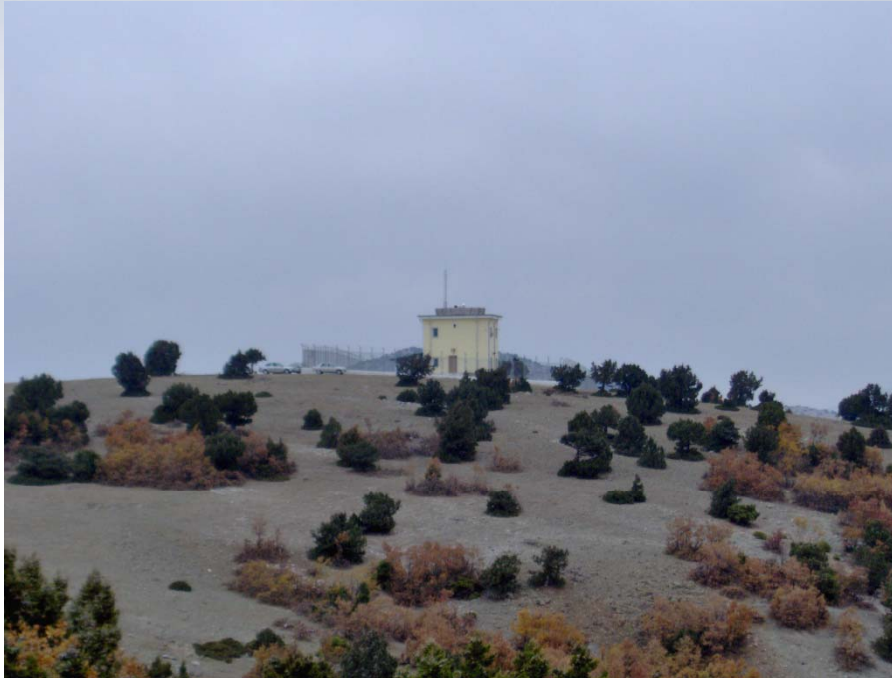
Transponder tower at western site
